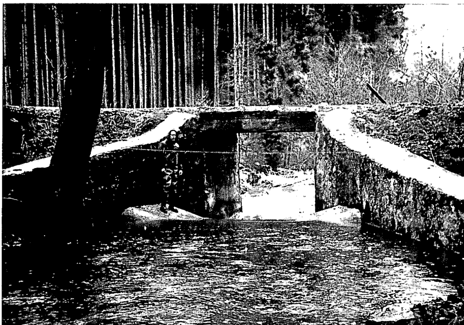
Photo 2 The side walls of the channel in which the weir is placed are not parallel
