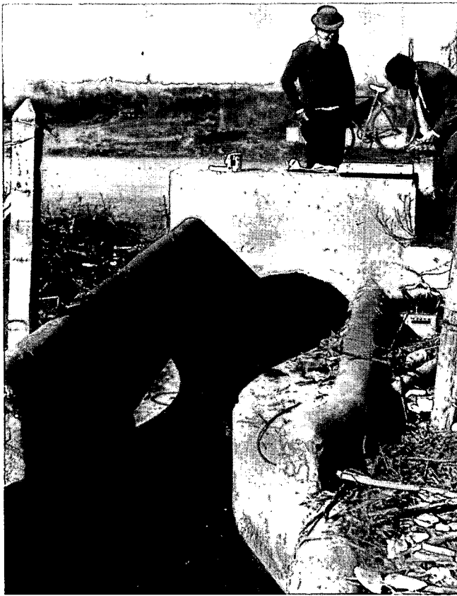
Photo 2 Throatless flume with rounded transaction
