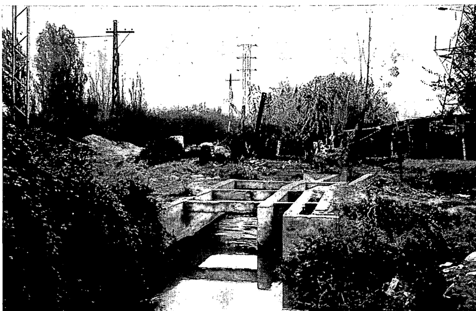
Photo 1 Proportional divisor with fixed pier in between the two weirs
